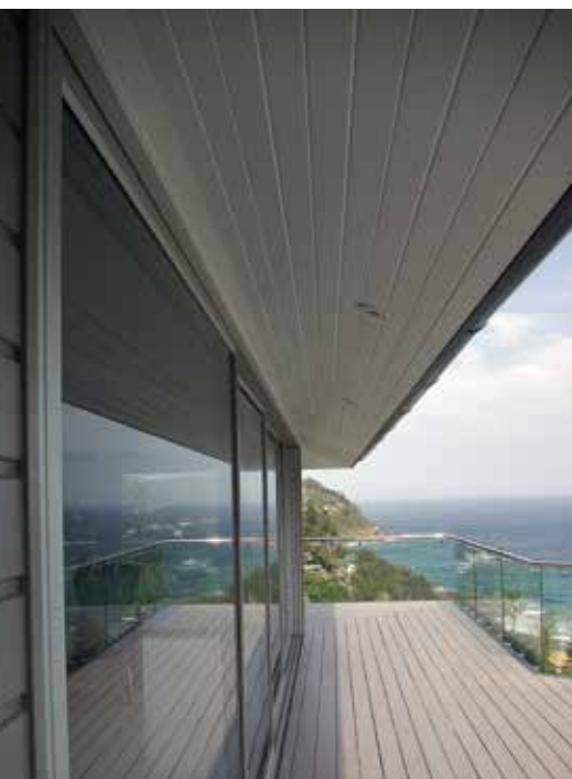
138 x 11 Vee joint eaves lining
