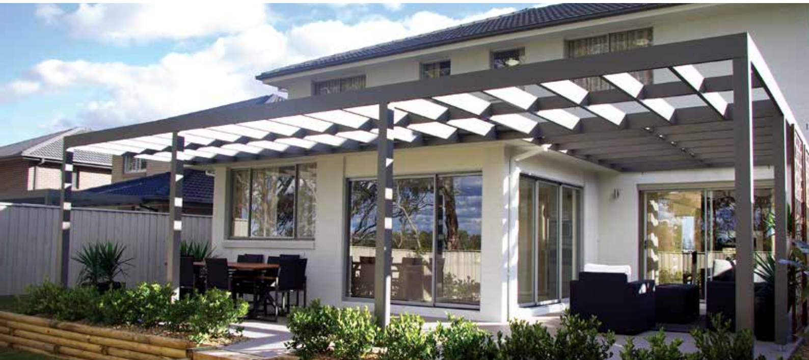
Posts, beams and rafters
