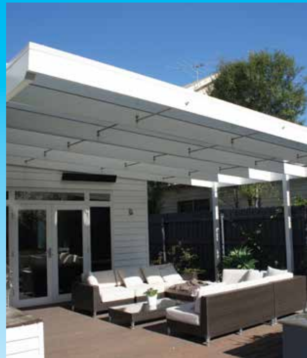
Posts and beams
